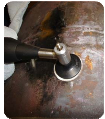
On-site grinding and polishing
